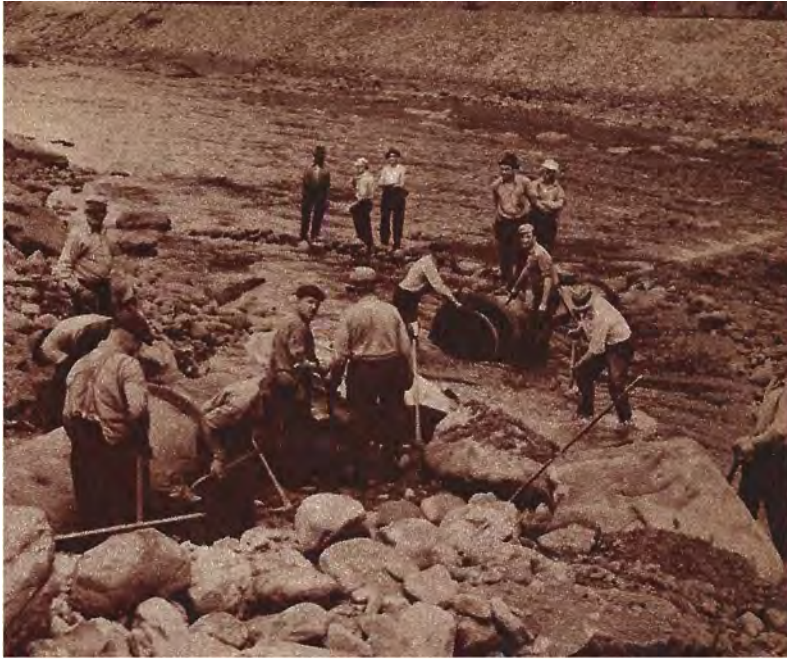
A dynamite explosion shattered the 36-inch water supply pipeline of the Cambria plant of the Bethlehem Steel Corporation. It caused a shutdown of the factory.
