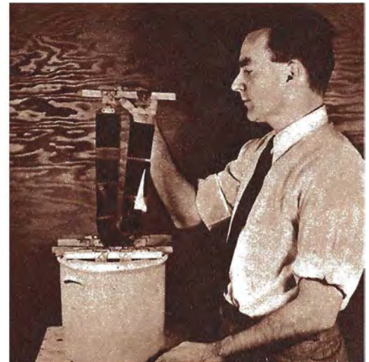
Below: Tray-developed cut or rollfilm may be fixed by suspension in a three-gallon crock full of acid hypo. Both ends of the rollfilm are attached to a stick laid across the top of the crock as shown. Lift and drain the film from time to time. The crock costs less than a deep tank and the system saves the usual see-sawing time.— Robert Scott.
