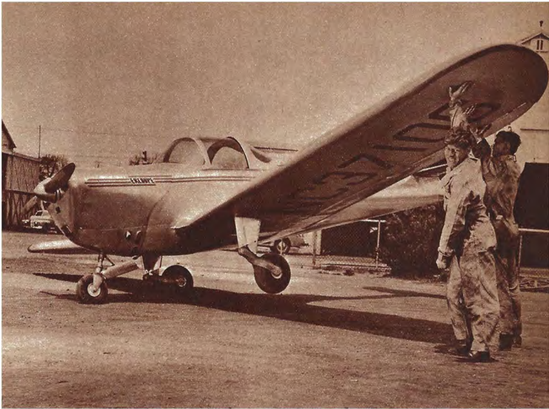
Here's how the landing gear compresses to absorb landing and taxiing bumps. It rides like an automobile.
